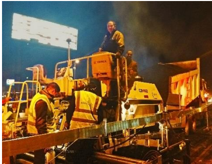
Jobsite at night: Cairo Motorway
